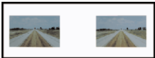
Slide #1 (2000-147) Demonstration Highway
